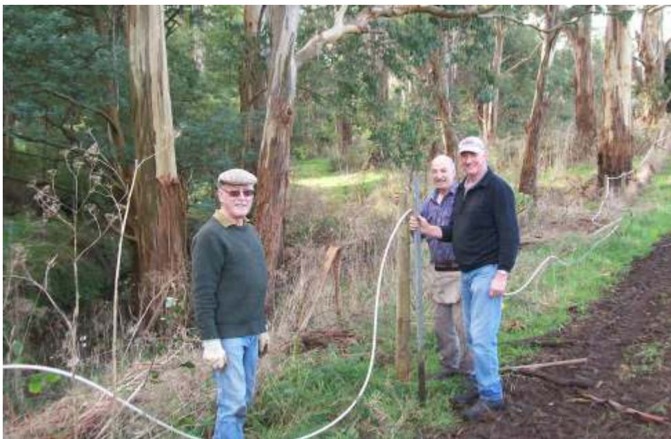
Korumburra Rotarians repairing the fence on the walking track which is now ready for use. Why not try it out. (see page 6 for details)
